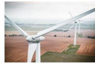
Sustainable Energy Solutions
