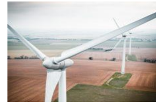
Sustainable Energy Solutions
