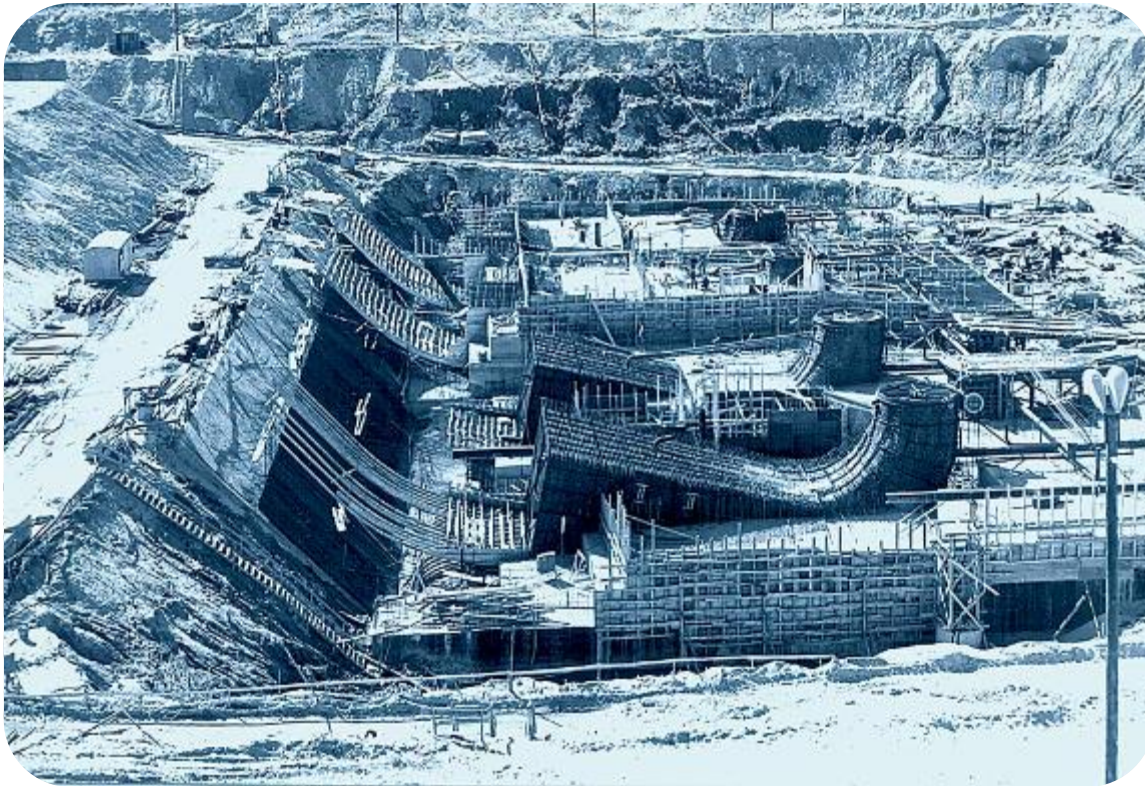
Fot. 1975 year – concreting suction pipes
