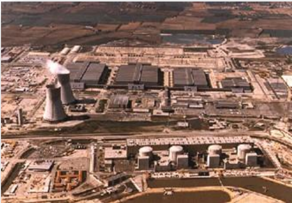
Fuel reprocessing plant, Marcoule, France
