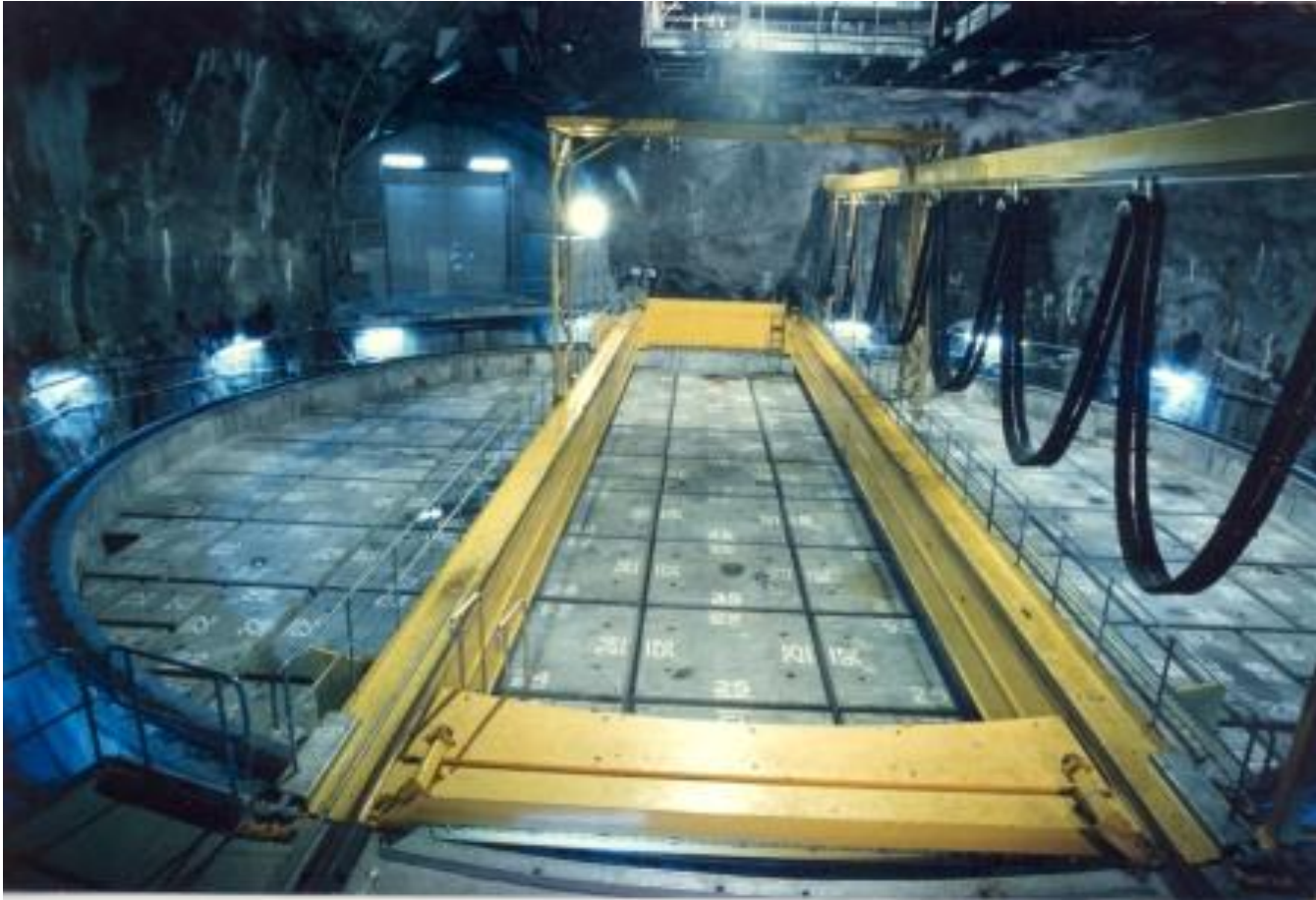
Landfill of intermediate activity waste (ILW) in Sweden (image: Bengt O. Nordin, Stockholm, Sweden, source: IAEA)
