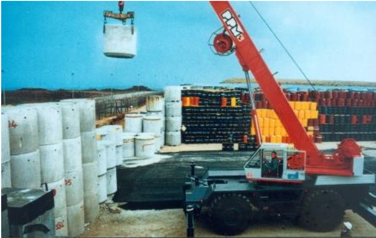
Landfill for low-level waste in the French region of France (photo: CEA, source: IAEA)
