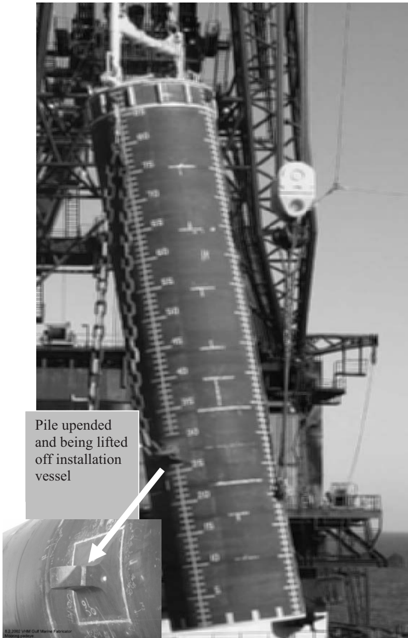
Fig. 2-13. A suction pile foundation for a spread mooring system as it is lifted
