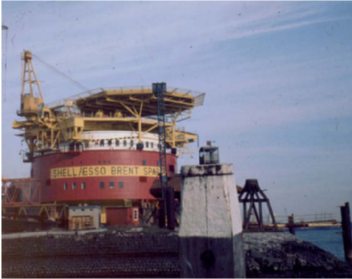
Fig. 1-1. Brent Spar under construction (Photograph courtesy of Quistnix)
