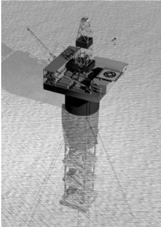
Fig. 1-16. Truss Spar (Courtesy of Technip USA, Inc.)
