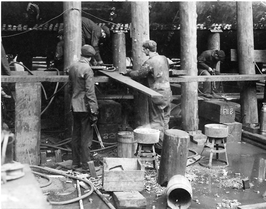
Photo # NH 44744 Riveters at work repairing USS Northern Pacific after she went aground, 1919
