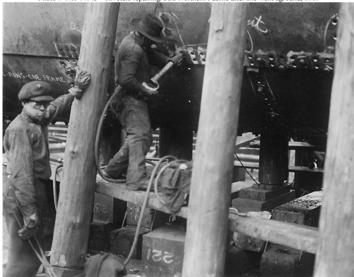
Photo # NH 44745 Riveters repairing USS Northern Pacific after she went aground, 1919
